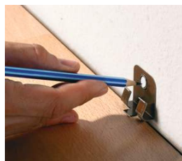
Align stainless steel clip and mark hole
