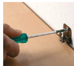
Align clip and screw in place
