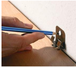
Align stainless steel clip and mark hole
