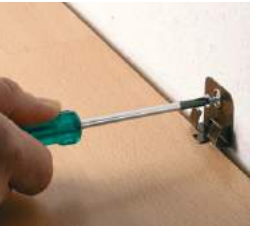
Align clip and screw in place
